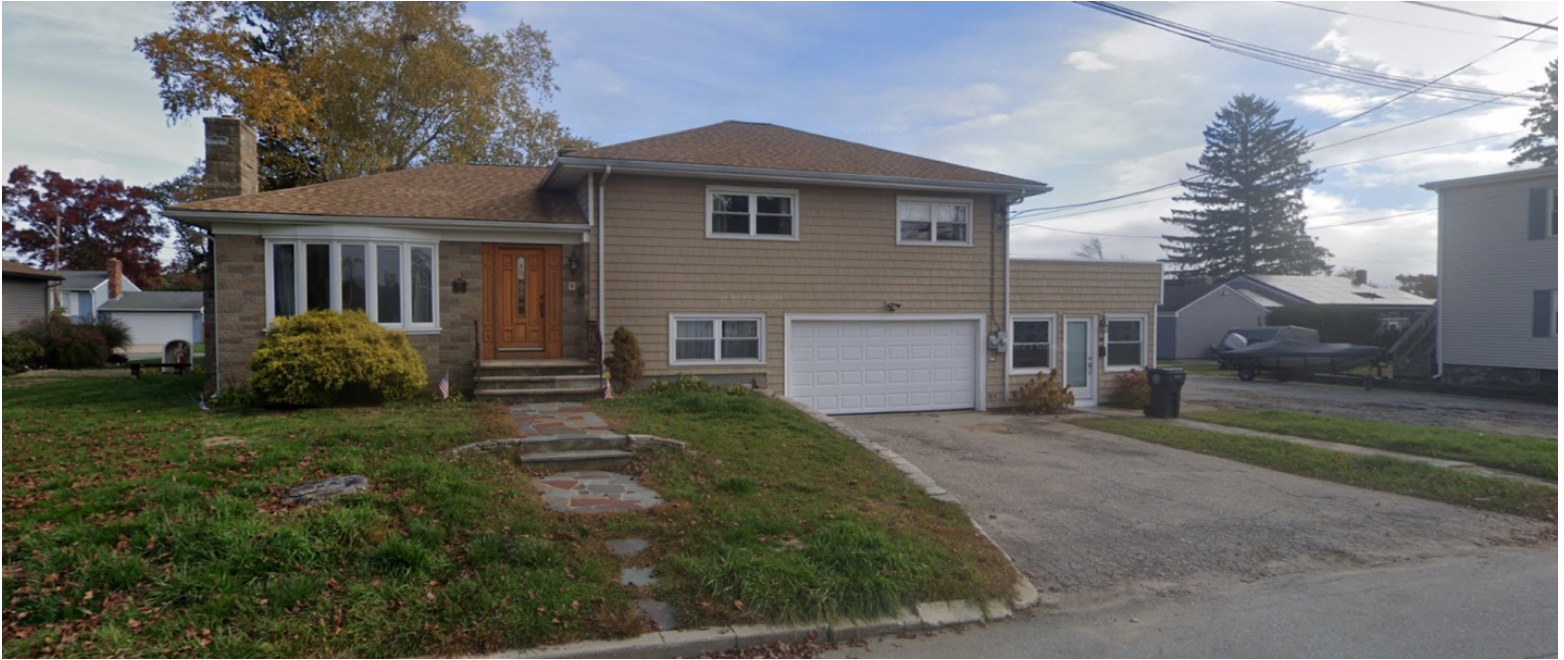
STREET VIEW (Kearney Street)
