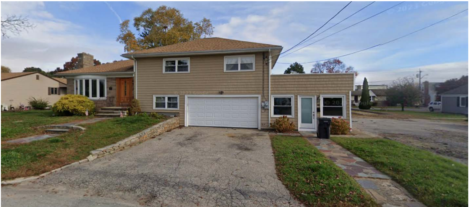
STREET VIEW (Kearney Street)
